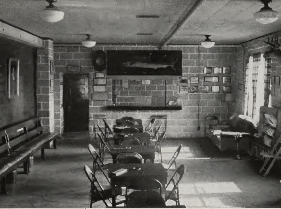
Above —Lightweight concrete masonry, exposed inside and outside, resulting in "a lot of good-looking building for the money". Recreation Hall and Auditorium, Eagle-Ottawa Leather Co., Grand Haven, Michigan. Robinson & Campau, architects.
